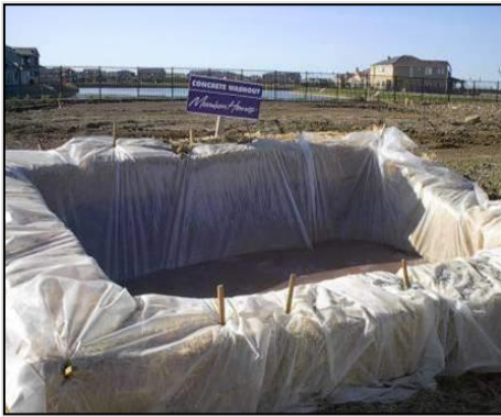
Plate 3-1 Typical concrete chute wash out areas
